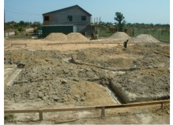
digging the trenches for footings
