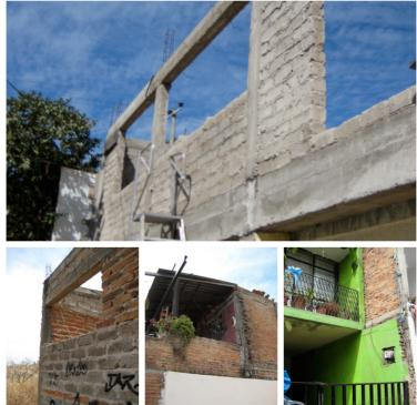
local building materials often consist of CMU or brick constructed with concrete columns and beams and brick infill
