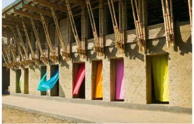
Ground level: The thick walls are formed in a local construction method out of mud work. Their construction allowed for local labor to be used and for the building to fit into the local context
