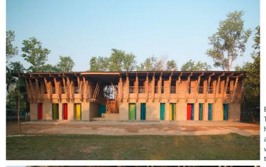
Exterior facade: The large overhangs help shade the building and prevent the mud walls from eroding in the rainy season.
