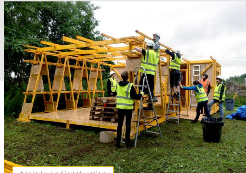
Main Build Construction
